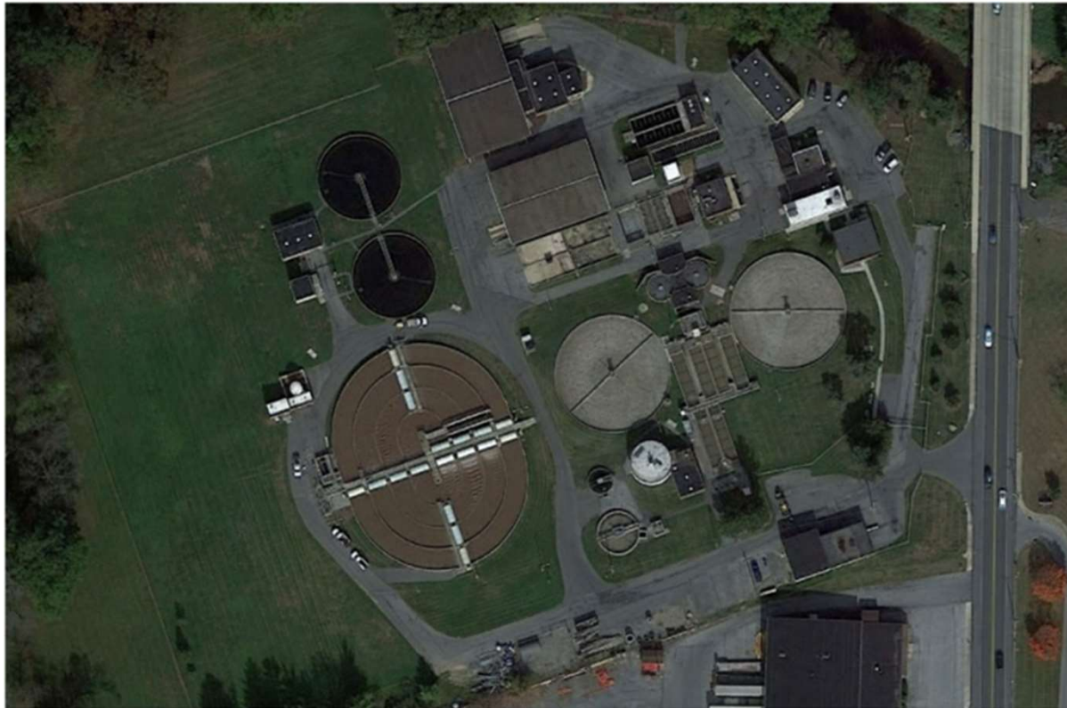
Figure 1 Ephrata Borough Authority WWTP #1
