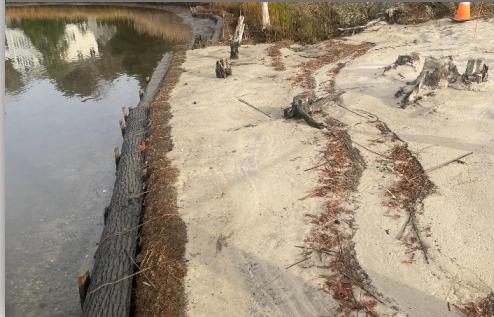
Living Shoreline Installation, Delaware
