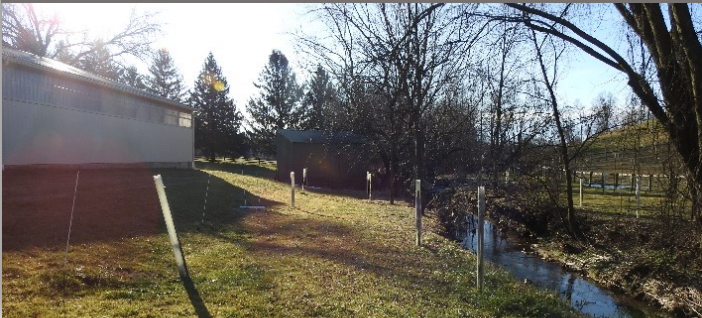
Micro Bio-Infiltration Swale, Pennsylvania
