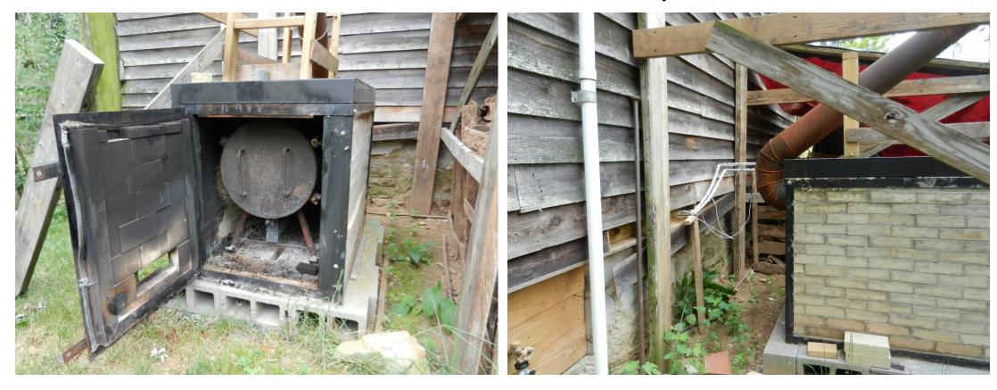
On the left is the production unit with the heavy piano hinged door open to show the firebrick insulation and the pyrolysis barrel inside. Note also the 12 cm high water tank that makes up the roof of the burn chamber. On the right is the back of the unit next to the house where the send and return pipes are seen. These are protected from the heat with reflective aluminum insulating tape.
