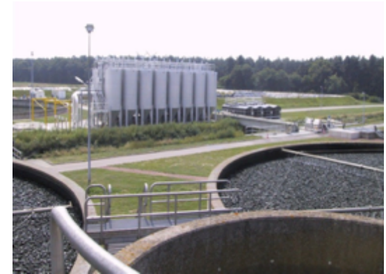
SLUDGE (Sewage, Digestat, Manure)
