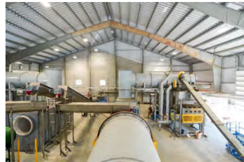
Bethel, PA Facility
